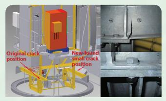
Figure 5. Internal space frame cracking
